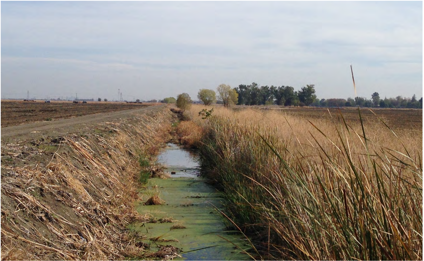
Existing Drainage Channel
